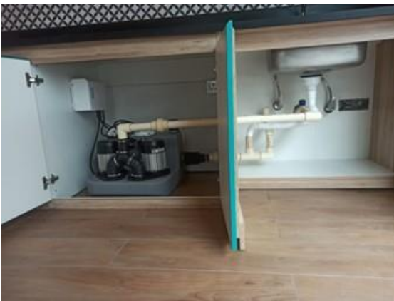
A Sanicom 2 connected to a kitchen sink under the counter.
