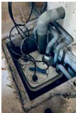
Sanicubic 1 WP installed in a pit
