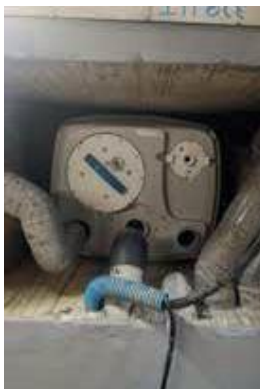
Sanicubic 1 VX installed in a pit
