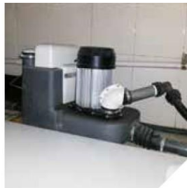
Sanicom 1 installed on the floor
